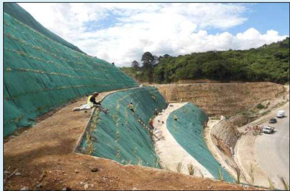
Very steep Batters with geofabrics (Leonel Castro)
