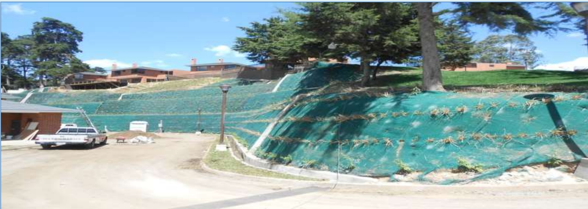
Very steep Batters with geofabrics (Leonel Castro)
