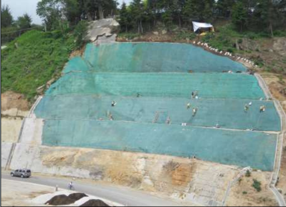
Very steep Batters with geofabrics (Leonel Castro)
