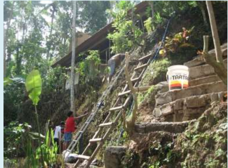
Planting vetiver using long ladders
